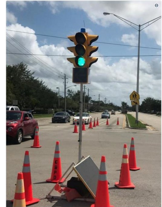
Temporary traffic lights in Coral Springs, FL
