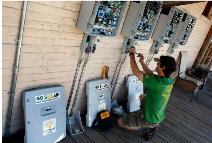
Installing solar potential
